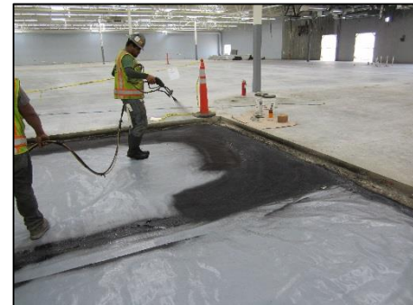
MTN Inc. union contractors apply Geo-Seal on-site.
